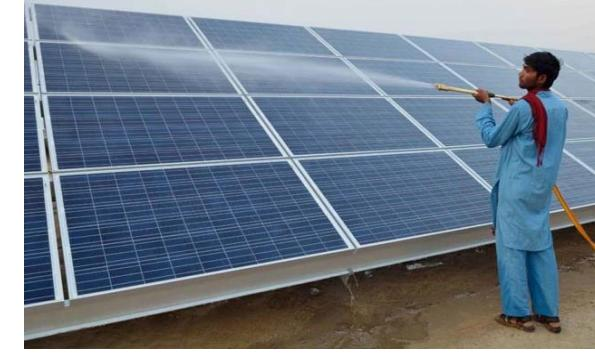
A photograph showing a person in a blue uniform and a red sash, using a long-handled cleaning tool with a spray head to clean a large array of blue solar panels mounted on a metal frame. The panels are arranged in a grid pattern, covering a significant portion of the ground. The person is standing on the right side of the frame, facing left towards the panels.
